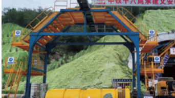
Yan'an-Yulin High-Speed Railway Wenanyi Tunnel
