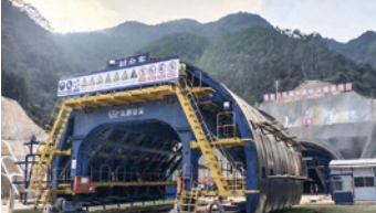
Puqing Expressway Lingding Tunnel
