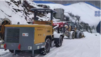
Shenyang-Baishan High-Speed Railway Shangshan Tunnel
