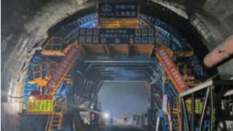
Chongqing-Hunan High-Speed Railway Zhangjiashan Tunnel
