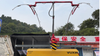
Shanghai-Chongqing-Chengdu Railway Pengbaoshan Tunnel
