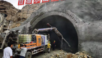
Baotou-Yinchuan High-Speed Railway Gandur Mountain Tunnel
