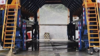
Sichuan-Tibet Railway Yigong Tunnel
