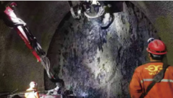
Sichuan-Tibet Railway Yingjinshan No.1 Tunnel
