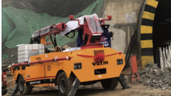
Wuxue-Yuxi Expressway Yangjialing Tunnel
