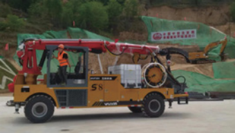
Pingliang-Qingyang Railway Fujiaping Tunnel
