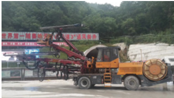
Baoji-Pingwu Expressway Qinling Tiantai Mountain Extra-long Tunnel
