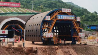
Sichuan-Tibet Railway Yigong Tunnel
