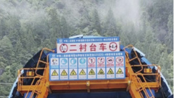
Xi'an-Shiyan High-Speed Railway Tianzhushan No.1 Tunnel
