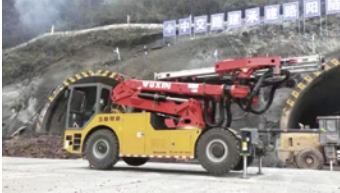
Wuxi-Yunyang-Kaizhou Expressway Luyang Tunnel
