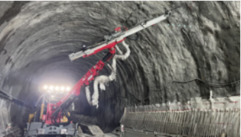
Malaysia East Coast Rail Link (ECRL) Project
