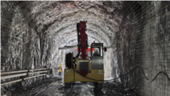
Jingning Pumped Storage Power Station Project
