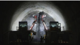
Leshan-Hanzhong Expressway Grand Canyon Tunnel
