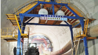
Chizhou-Huangshan High-Speed Railway Tiesiling Tunnel
