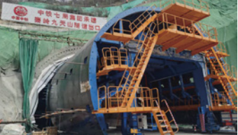
Xi'an-Ankang High-Speed Railway Qinling Jiutianshan Tunnel
