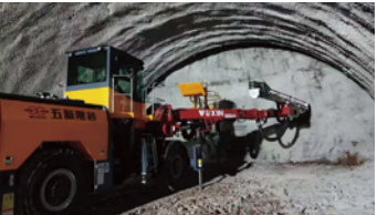
Chongqing-Guizhou Expressway Parallel Line
