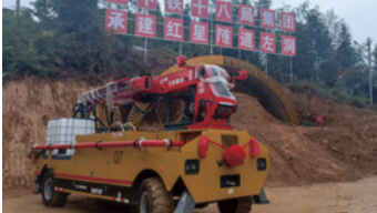
Suiichuan-Dahe Expressway Hongxing Tunnel
