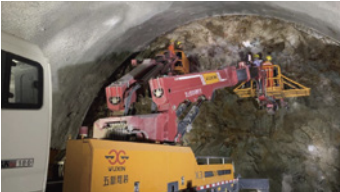
Jiumian Expressway Baima Tunnel
