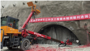
Yangtze River-Han River Water Diversion Project Water Conveyance Tunnel
